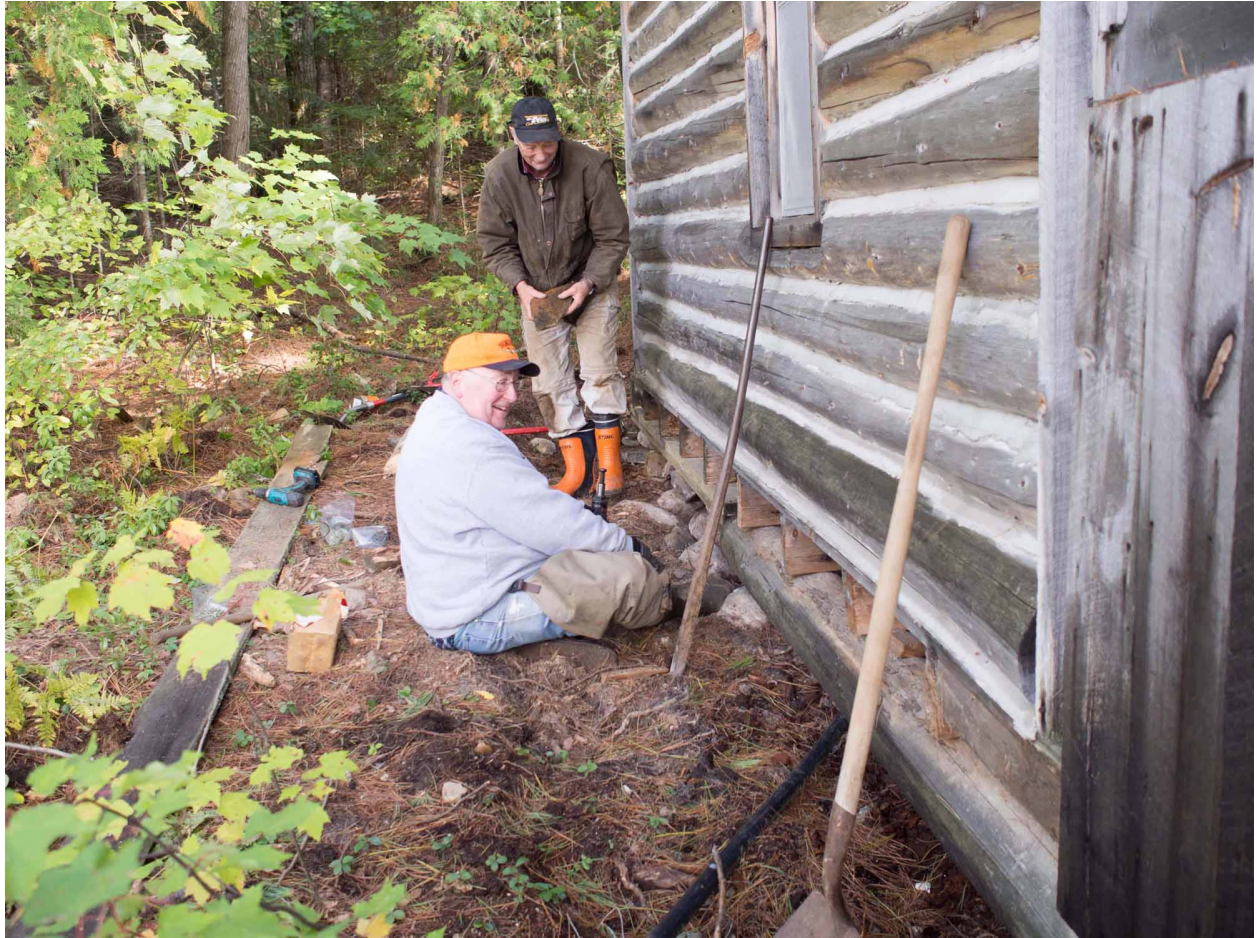
Roger and Dick replacing sills at Lost
